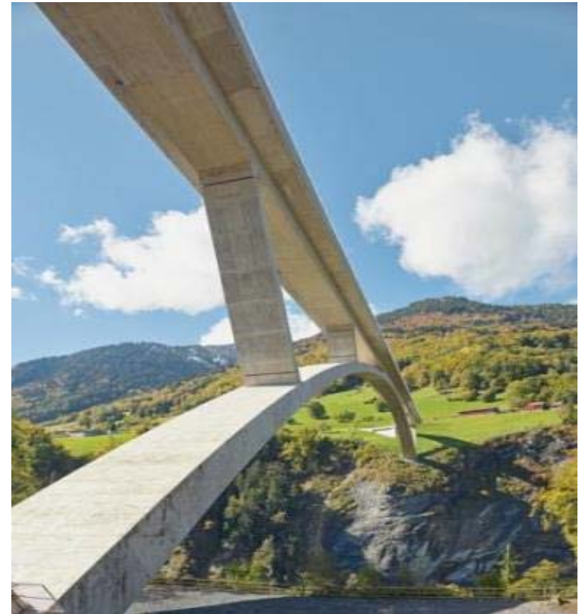
Tamina bridge - Switzerland
